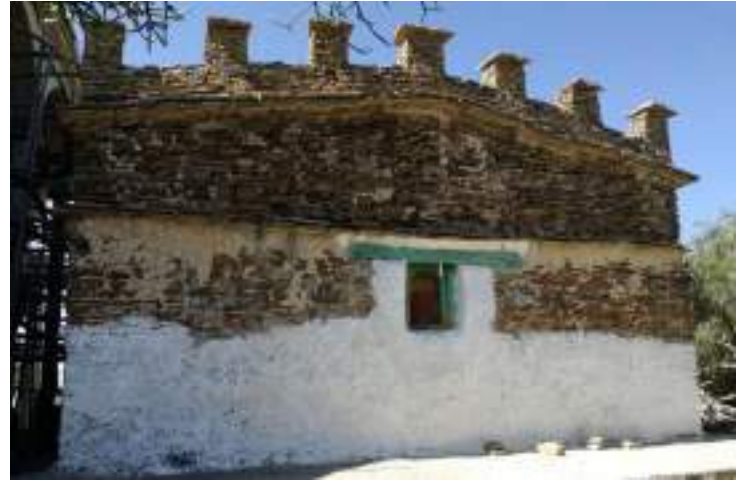
Fig. 10: The eastern outer wall of the 19th century church and the bay-window of the choir.
