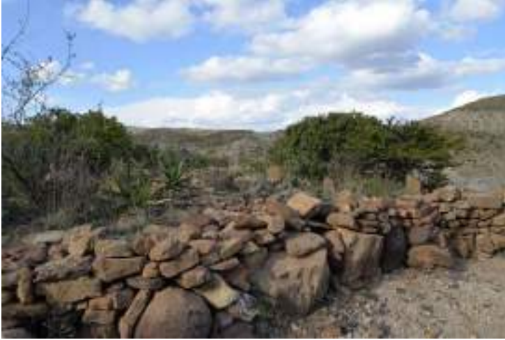
Fig. 66: Detail of the enclosure's wall.
