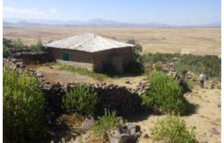
Fig. 20: The mosque in its enclosure with its protruding semi-circular mihrab.
