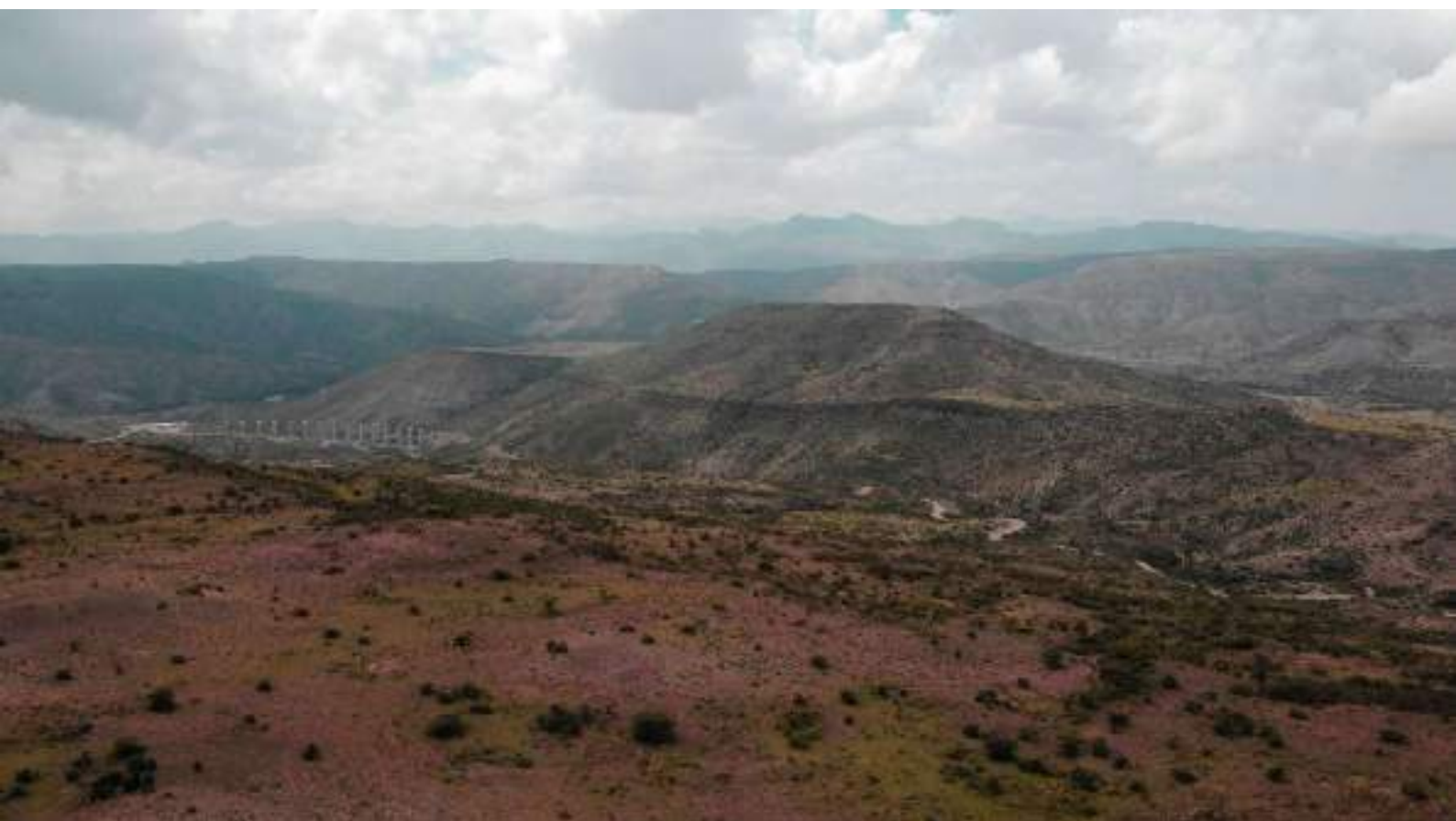
Fig. 93: The view from Habera toward the south. Note the railway bridge under construction to the left.
